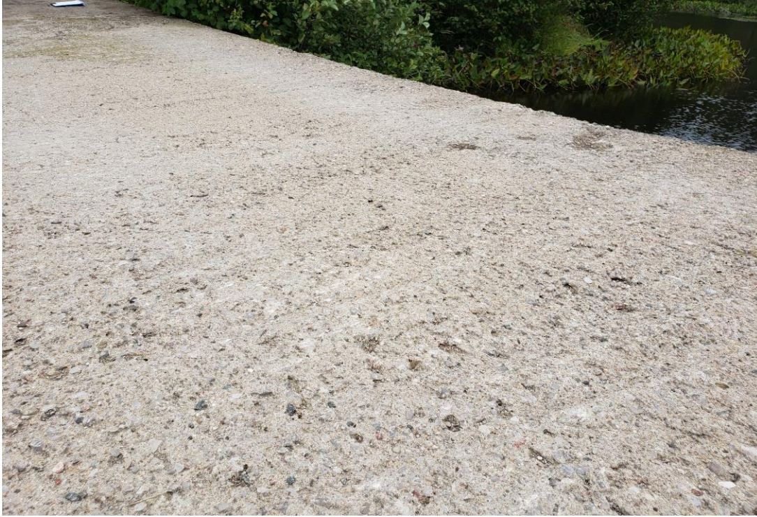
Description of Photo: Photo 6 - Bridge Wearing Surface.jpg
