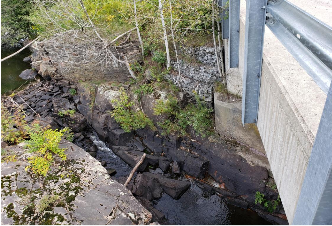
Description of Photo: Photo 34 - Gabion Baskets.jpg
