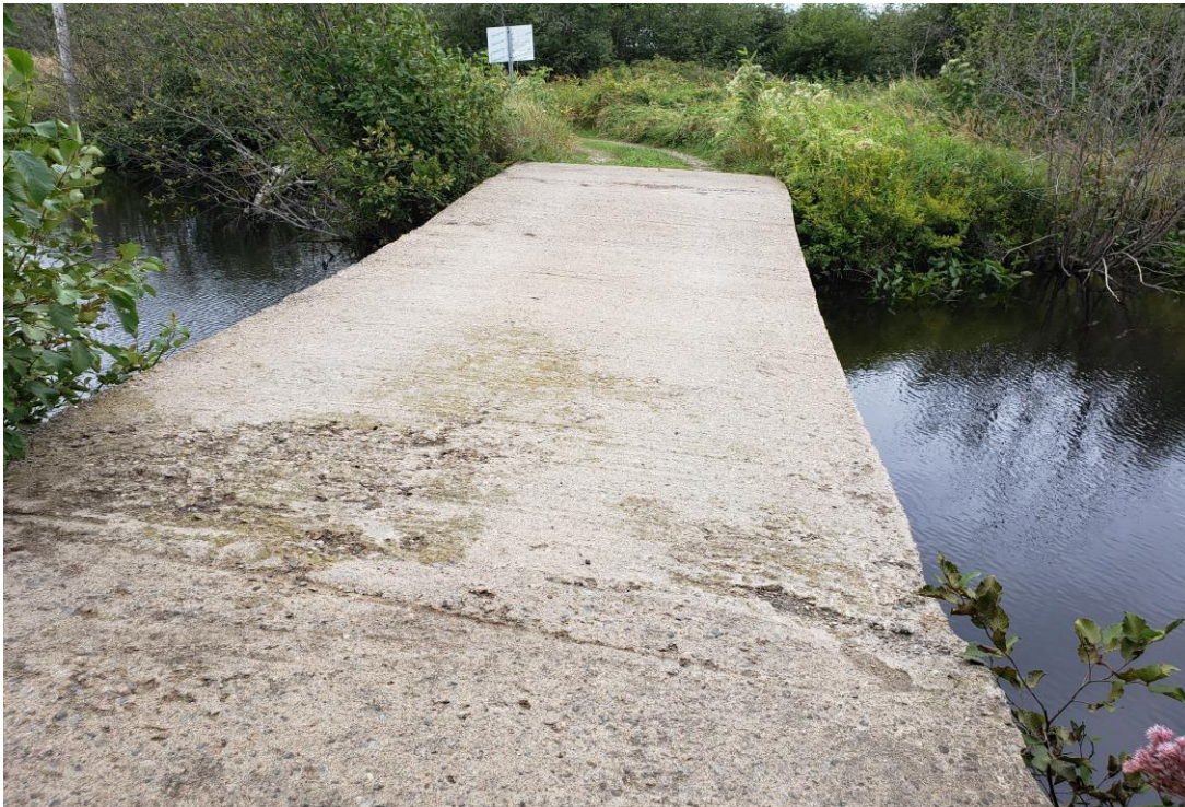
Description of Photo: Photo 7 - Bridge Wearing Surface.jpg
