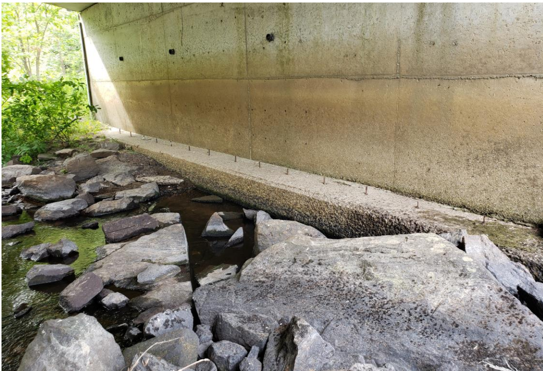
Description of Photo: Photo 41 - Rock Protection.jpg
