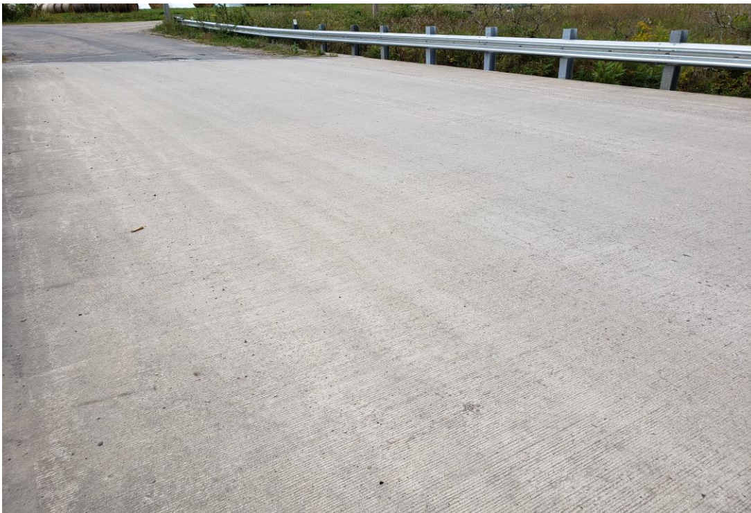
Description of Photo: Photo 14 - Bridge Wearing Surface.jpg
