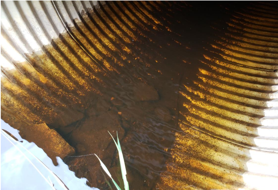
Description of Photo: Photo 17 - Overflow Culvert.jpg
