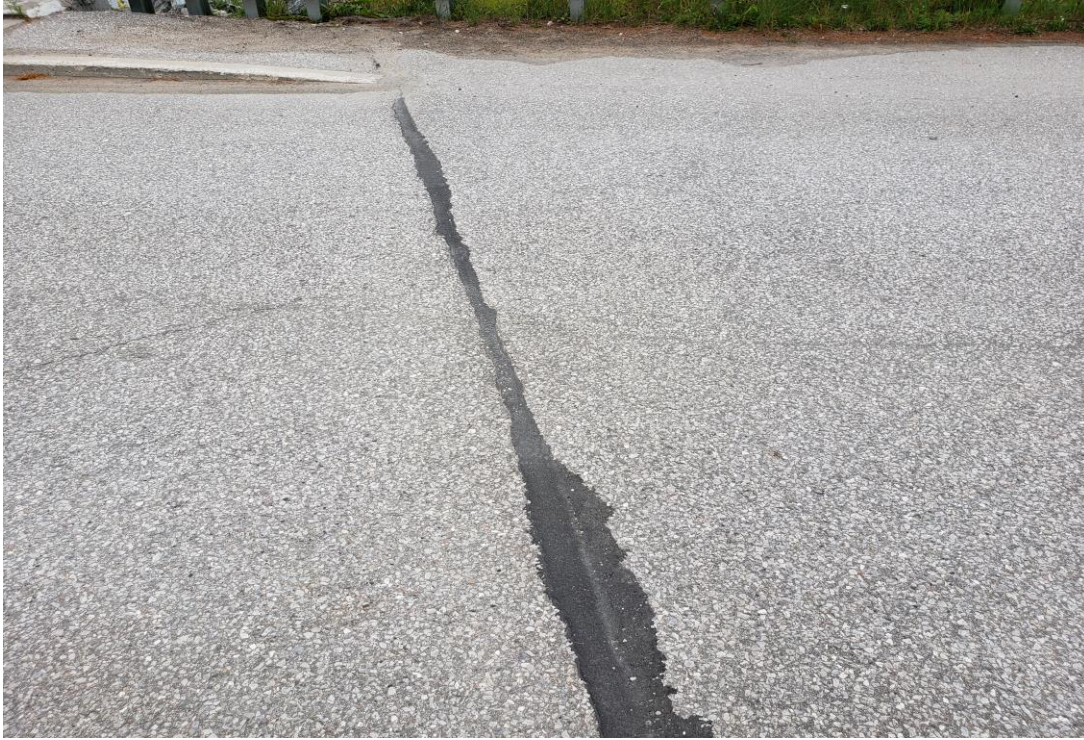
Description of Photo: Photo 18 - Seal.jpg
