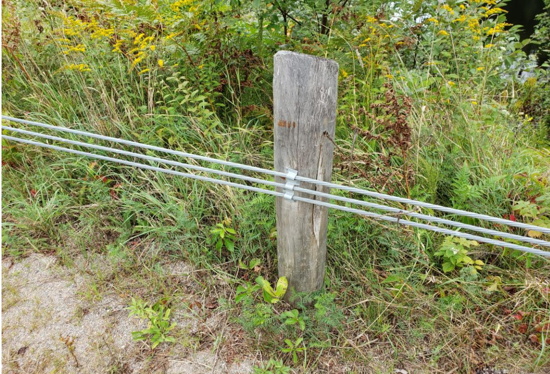
Description of Photo: Photo 7 - Approach Barrier Post.jpg
